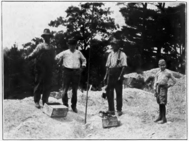
Tamping Charge of Dynamite in the Drill Holes at Lewiston. Mr. Martin, head of the Company in the Straw Hat
